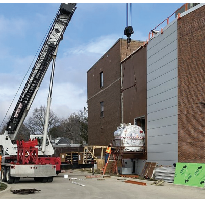
The 16,000 pound magnet is lifted into the building.
