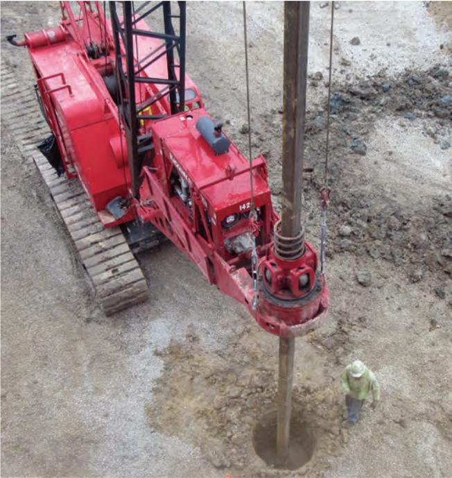
Pier drilling begins for the rebar cages. Over 50 holes were drilled ranging from 30-50 feet deep.
