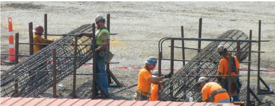
Iron workers construct cages made from rebar to be used to support the foundation of the new addition.
