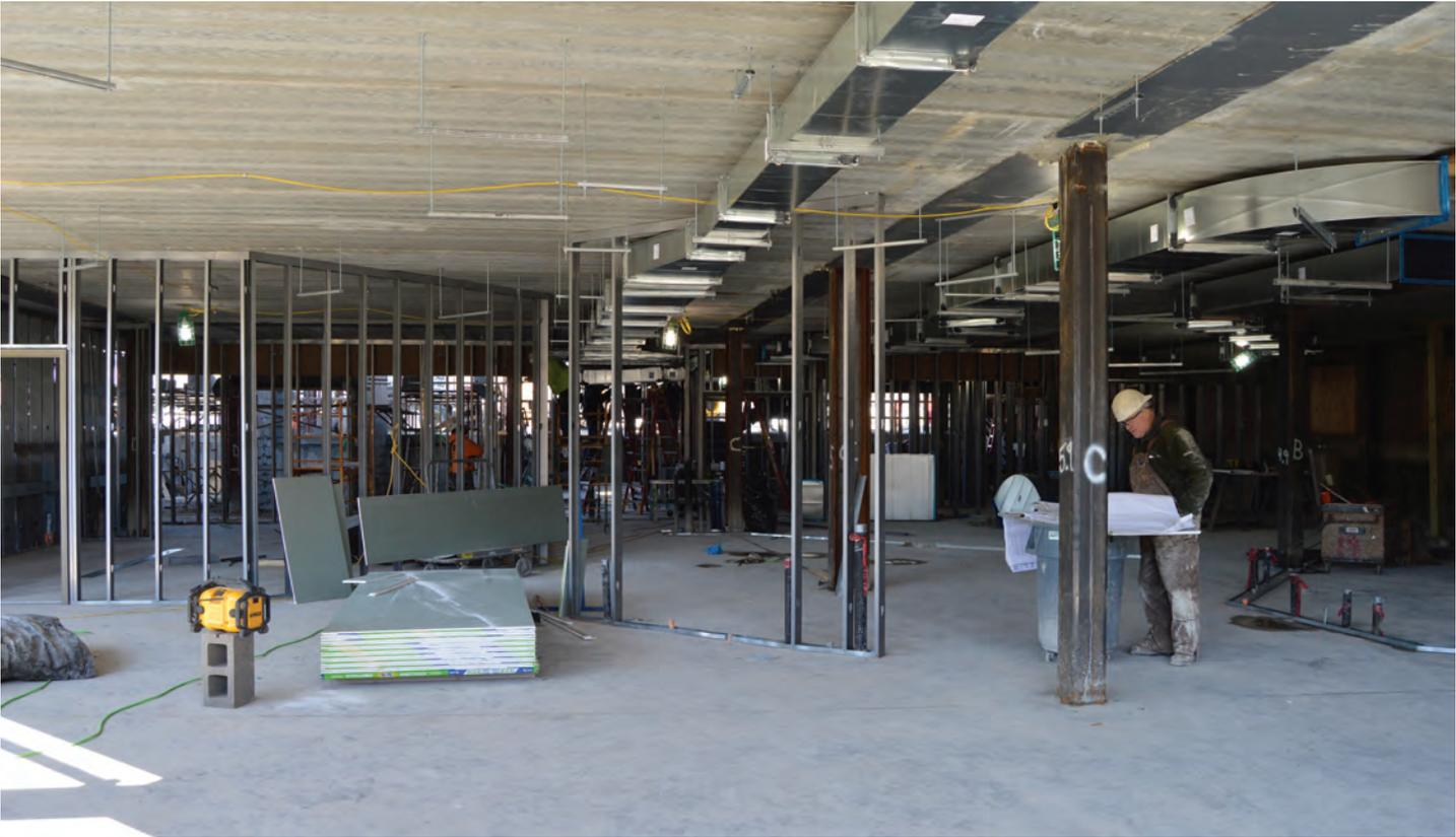
Above: Interior duct work and walls are constructed.
