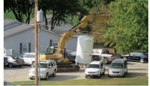
The oxygen tank had to be relocated to make room for the patient services addition. Here the oxygen is released and tank is moved.
